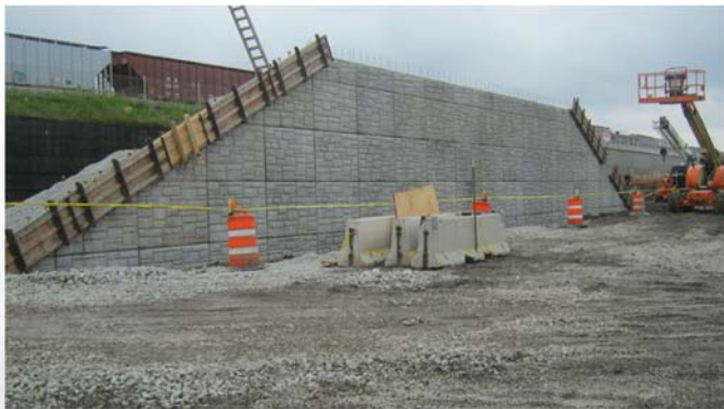
Construction of retaining wall
